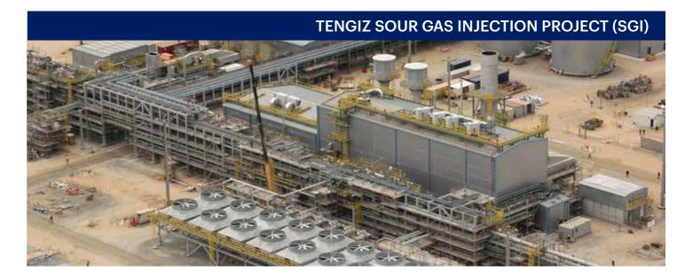
Installed a compressor and associated piping systems capable of delivering sour gas (17%  $H_2S$ ) into the reservoir at 10,000 PSI ,
