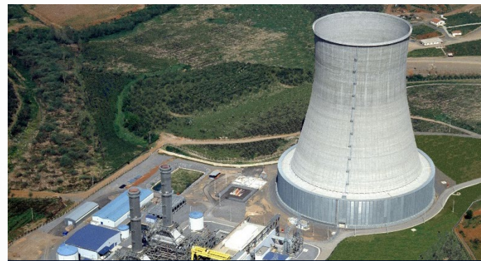
ADAPAZARI NATURAL GAS FIRED CCPP 820 MW
