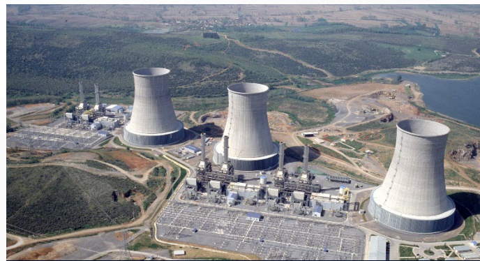
GEBZE NATURAL GAS FIRED CCPP 1,600 MW
