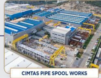
ÇİMTAŞ PIPE SPOOL WORKS
