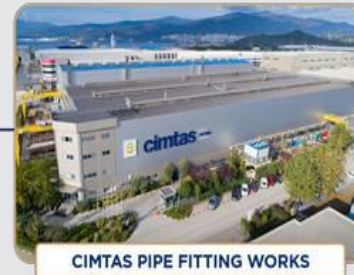
ÇİMTAŞ PIPE FITTING WORKS
