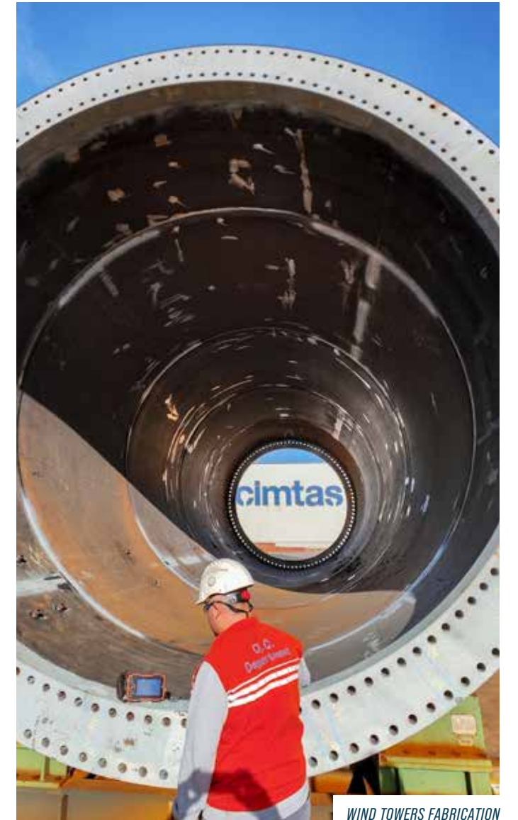
WIND TOWERS FABRICATION
